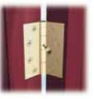
A front door that opens outward has hinges accessible from outside. To make them impossible to remove, flatten both ends of the pins or insert a screw in the center that is impossible to remove.
