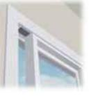
Patio doors can be lifted and removed without much effort. Install a plate or screw in the upper track.
